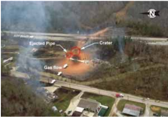
Figure 2. Pipeline Accident in West Virginia [5]
